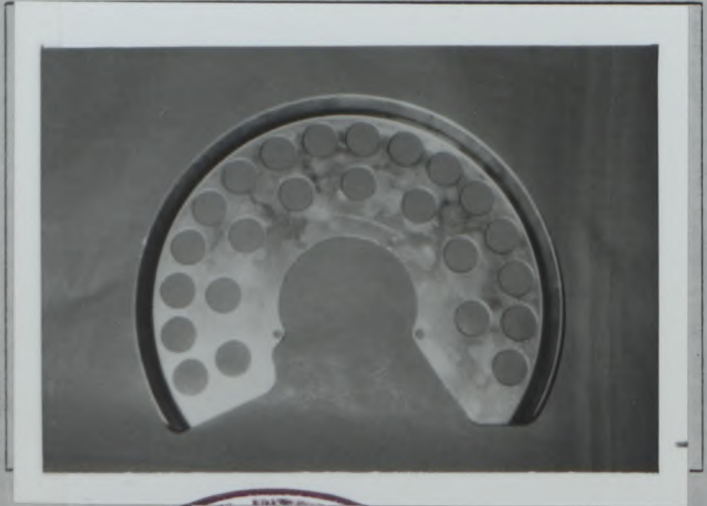
Photo Z34 Dust shield, brake
